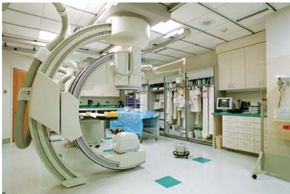
Cardio Vascular Lab Renovation
