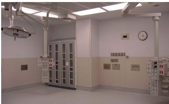
Operating Room Renovation
